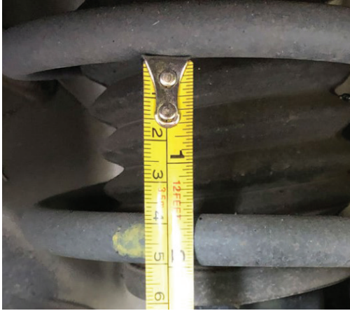
1. Due to the tight fit, top inner ring was cut off for easier installation process
